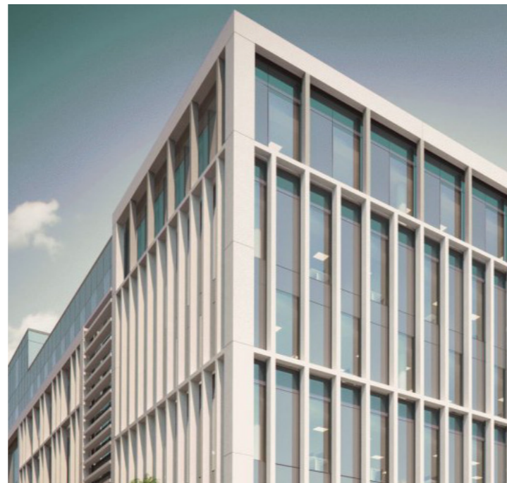
FIG 87 White stone cladding
