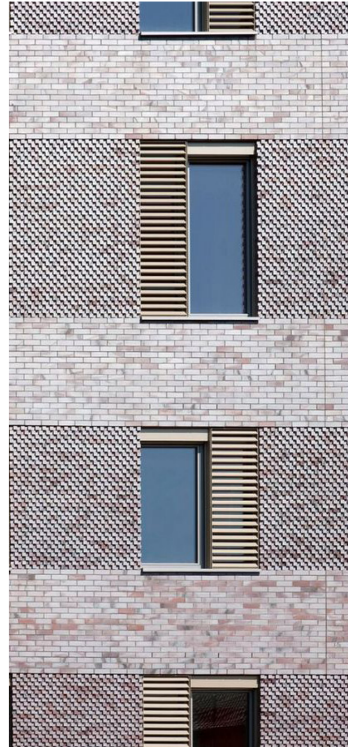
FIG 77 Articulated brick detailing
