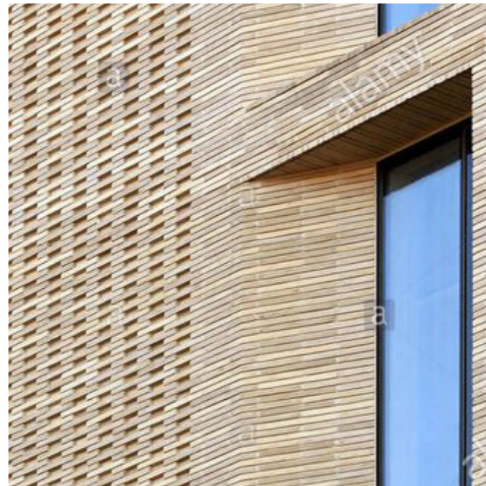
FIG 79 Sample of rusticated brick detailing
