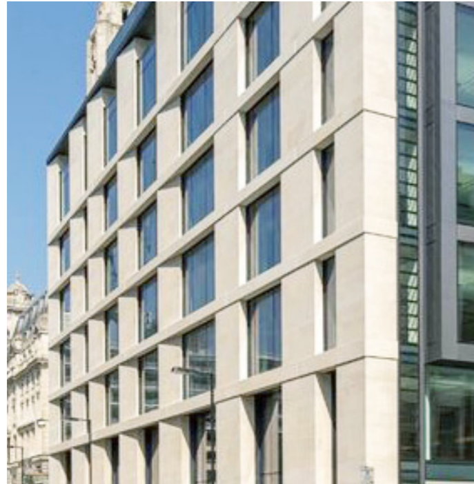
FIG 84 White stone cladding
