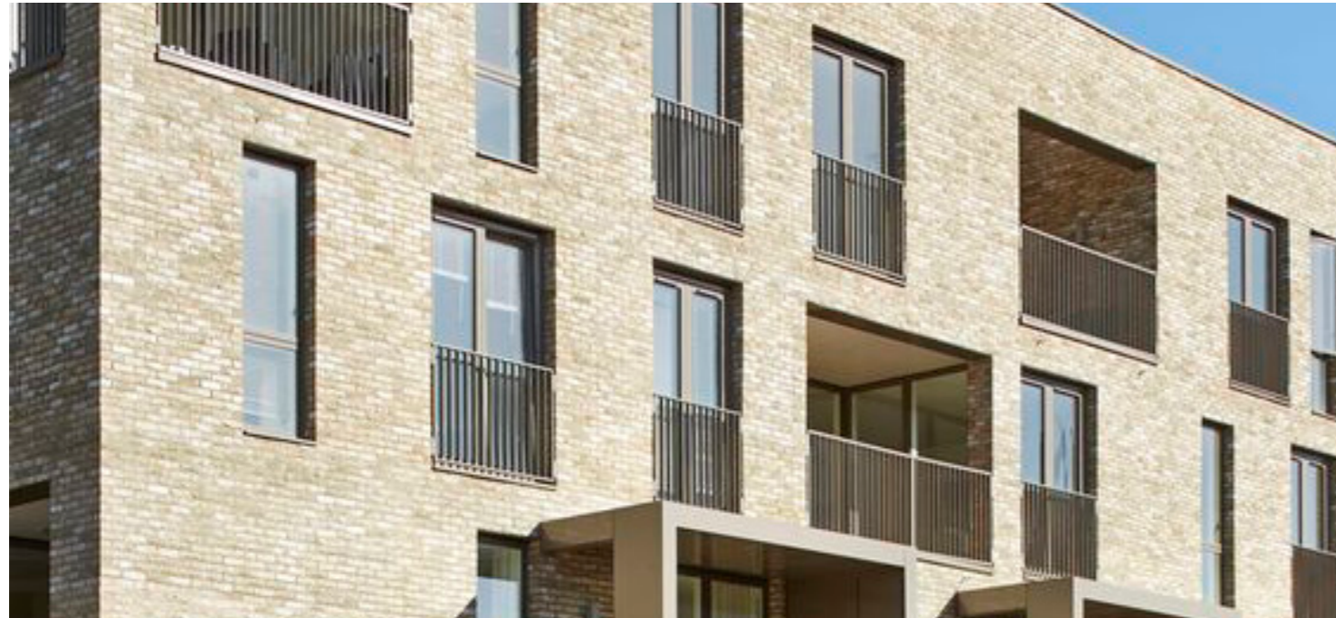
FIG 74 Brick facade with metal balconies
