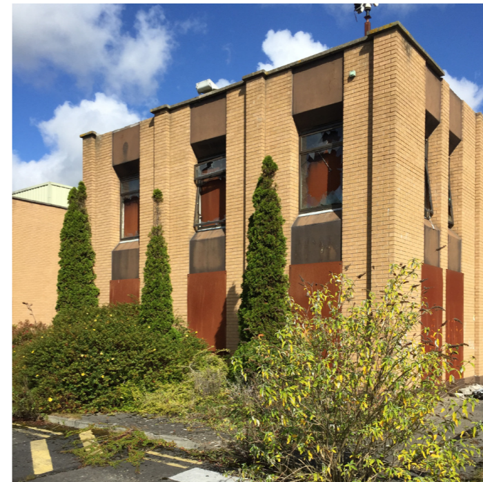
FIG 19 View of existing buildings on site
