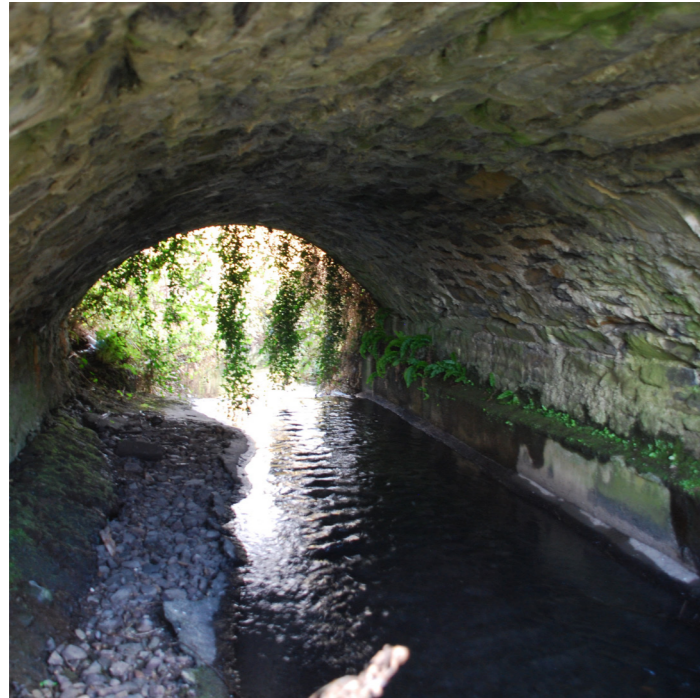
FIG 14 View under existing bridge over Santry River
