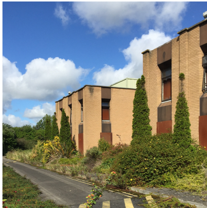
FIG 18 View of existing buildings on site
