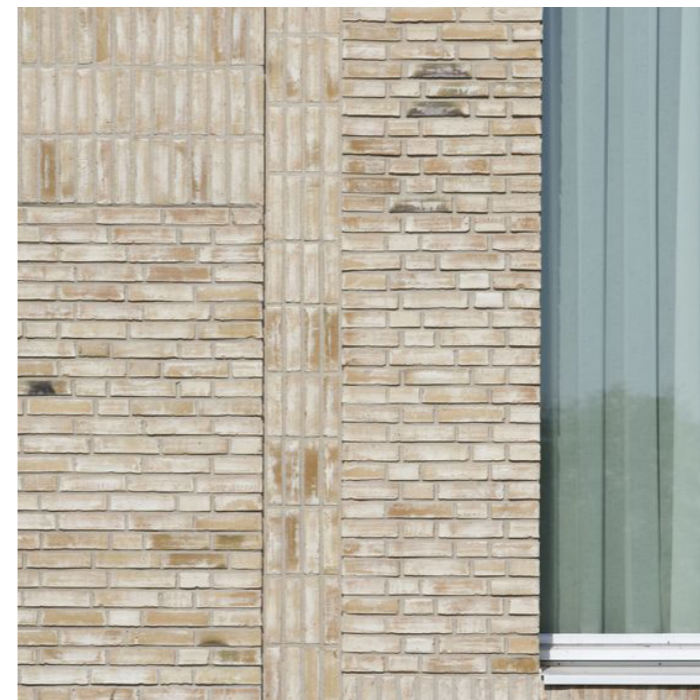
FIG 83 Sample of rusticated brick detailing
