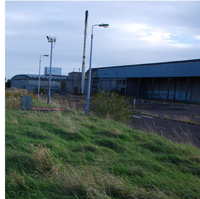
FIG 16 View of existing buildings on site
