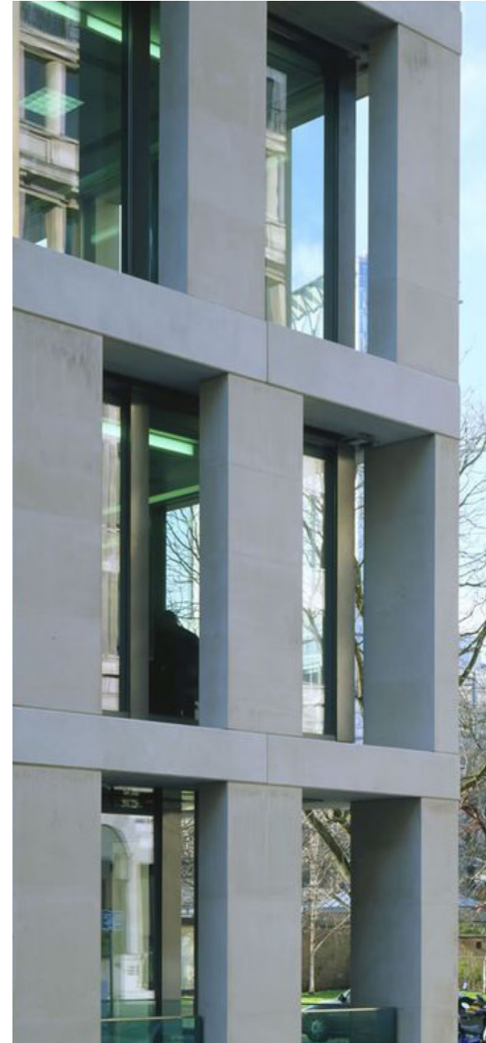
FIG 88 Regular openings in stone panel cladding
