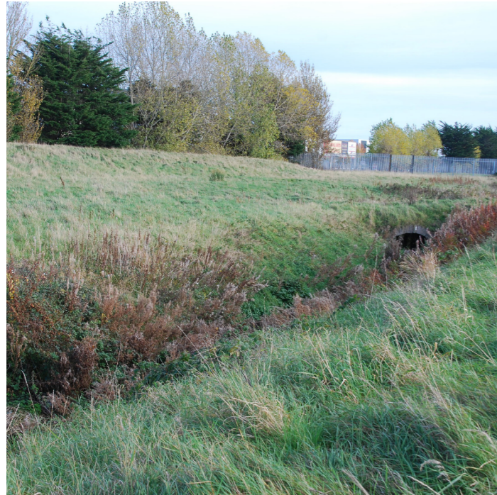
FIG 8 View of existing bridge over Santry River
